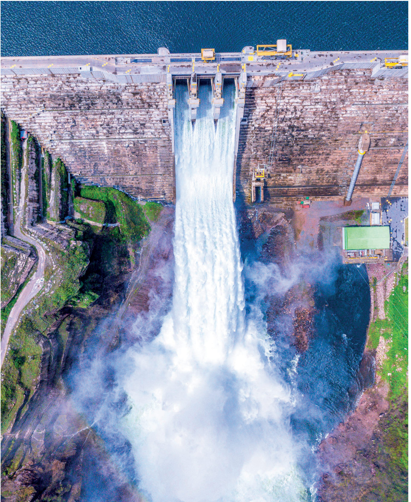
The Laúca Hydroelectric Power Station, Angola
